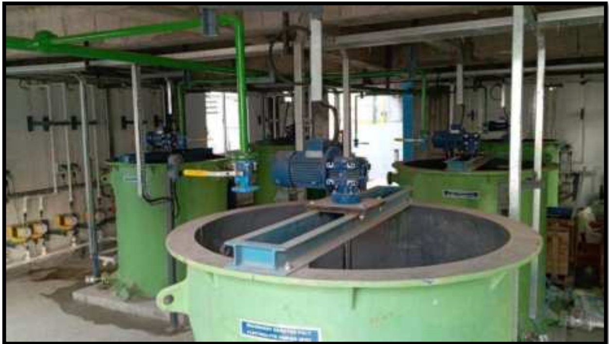
CHEMICAL DOSING SYSTEM, PSF & ACF
